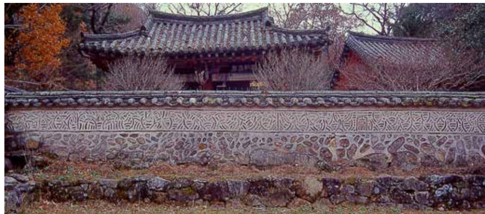
Wall at a Buddhist temple, built with roof tiles, white mortar and stones photo - Chung Hyun Cho, 1980
